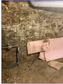
Foundation walls view.
