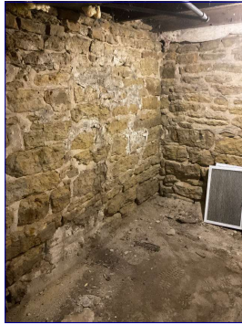
Foundation walls view.
