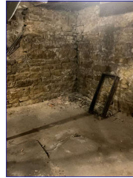
Foundation walls view.
