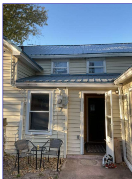
The Roof View
