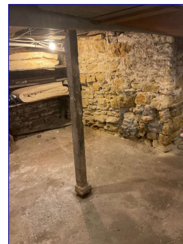
Foundation walls view.
