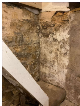
Foundation walls view.
