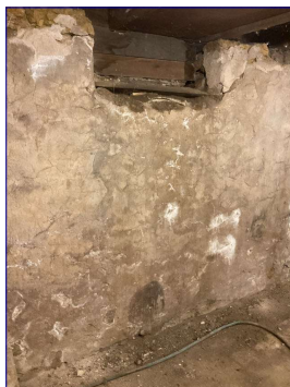
Foundation walls view.
